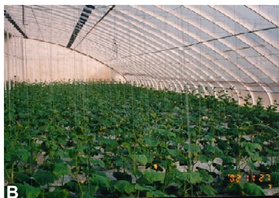
Fig. 3 Improvement on SPG framework. (A) bamboo and wood structure with concrete columns; (B) solid steel framework without support columns.
