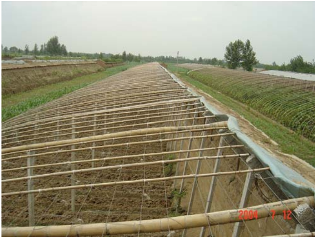
Fig. 2 A SPG with bamboo arch struts and concrete support columns.
