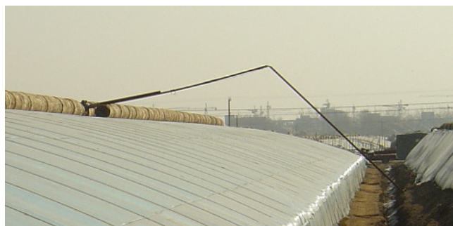
Fig. 6 Rolling up or releasing the thermal insulation curtains by machine.
