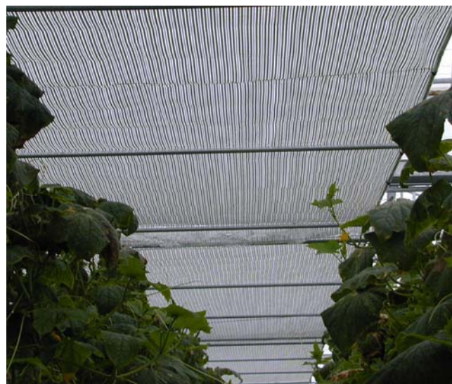
Fig. 3 Thermal screen used for energy saving and greenhouse shading.
