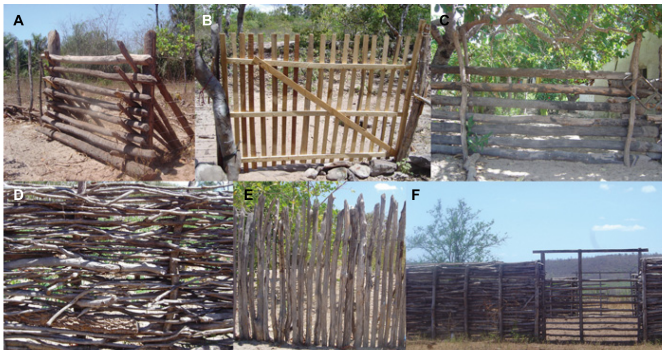
Fig. 2 Fences and gates used by the population of Cocal County, Piauí, Brazil. (A) Porteira , (B) gate, (C) passageway fence (fence of passagem ), (D) fence of cama , (E) fence of fachina , (F) barbed wire fence.
