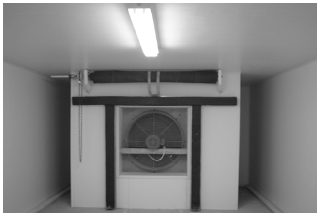
Fig. 2 Forced air cooler tunnel type.
