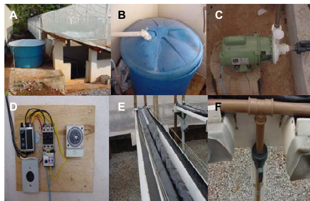
Fig. 4 Structure of the NFT hydroponic unit installed at the Universidade Federal de Lavras for the cultivation of seed potatoes from cvs. 'Monalisa' and 'Ágata'. The green house (protected with anti-aphid netting) and the reservoir of nutrient solution (2000-5000 L) are close to each other (A). The pump and the small tank of nutrient solution (2000 L) are inside the pump house (B). The pump, placed below the level of the tank, is covered with PVC (C) and attached to the control unit and timer (D). The cultivation channels (E), supported by wooden benches, are 4 m long and receive the nutrient solution through tubes connected to the pump (F). Photos: Ricardo Monteiro Corrêa.
